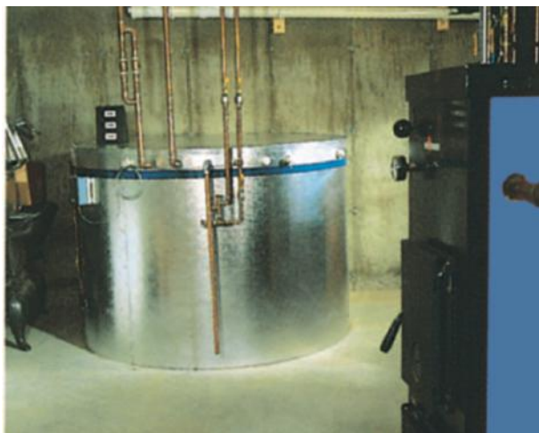
HS-TARM boiler with Heat Storage System.
