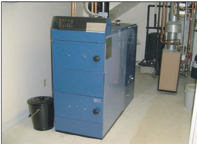
Multi-Heat: Fully automatic stoker boiler with hopper
