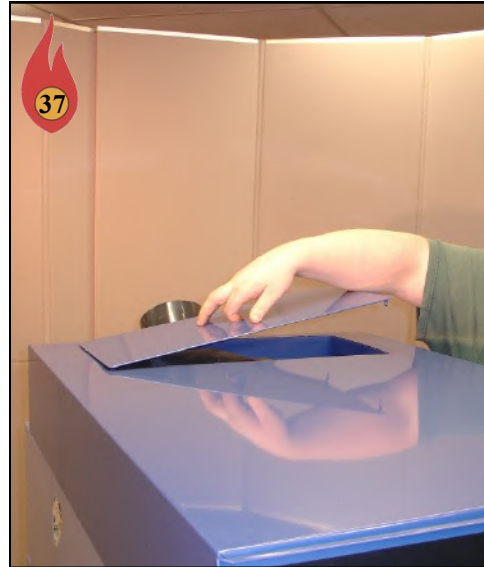
Place Clean-out cover lid over the Clean-out Opening. Bend the 4 tabs on the Cover in the Downward Position
