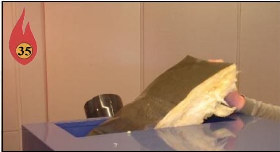
Place Insulation over Clean-out Cover (Removed Earlier)
