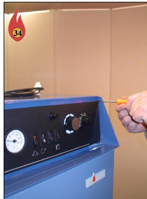
Fasten Control Panel
