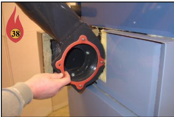
Place Fan Gasket on Housing
