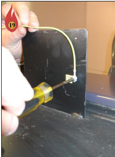
Install Ground Wire for Control Panel
