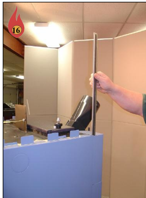
Install Right Rear Corner Zip Strip
