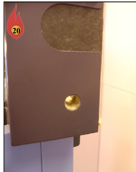
Remove Insulation for Lo-Limit Temperature Probe on Fan Insulation Box
