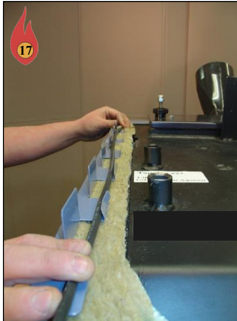
Place Power and Control Wires In Side Wire Channel
