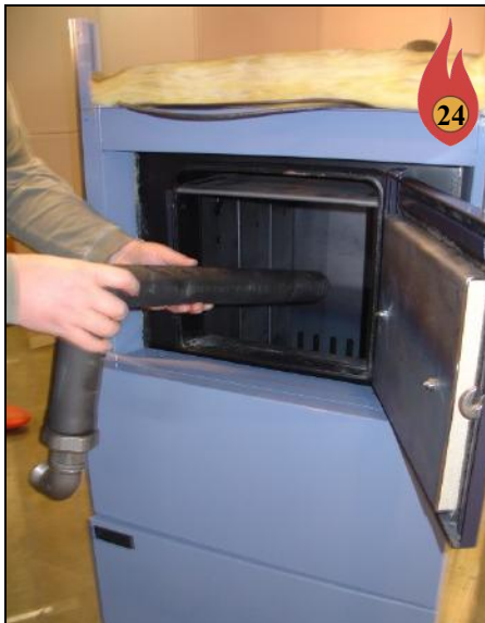
Remove Supply Pipe Assembly from Boiler
