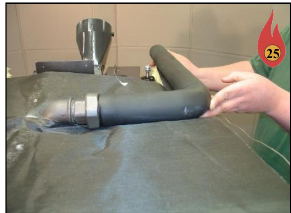
Install Supply Pipe Assembly. It can be Installed on the Right or Left Hand Side.
