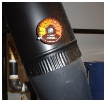
Fig. 3.5 339N Thermometer Installed
