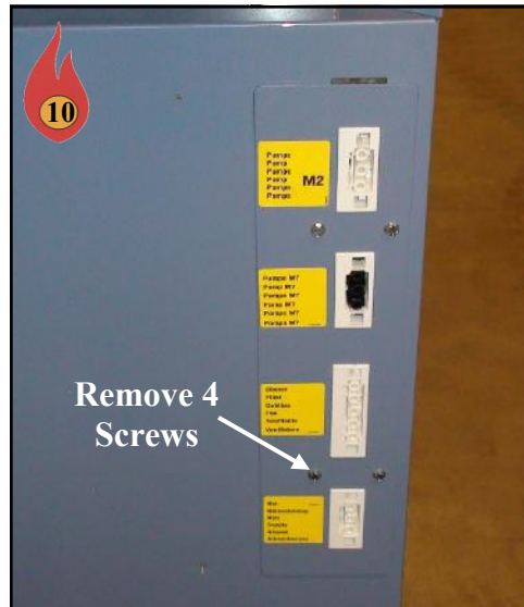
Remove the connector panel and wire harness on the back of the boiler by removing the four screws.
