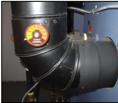
Fig. 3.5 339N Thermometer Installed
