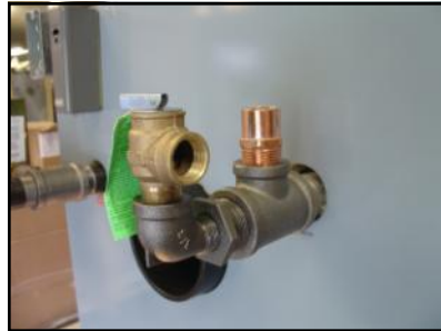
Fig. 3.6 Installed Relief Valve
