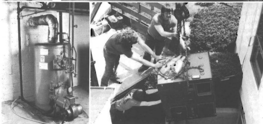
Multifuel unit (top) operates at efficiency of 84 percent (oil) or 62 percent (wood). Old oil burner (below, left) was 68 percent efficient. Door and unit sizes were compared before boiler was delivered. Basement entry eased task of getting new unit in, old one out.
