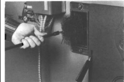
Wire flue brush and long-handle scraper were provided with unit for cleaning creosote from inside boiler.
