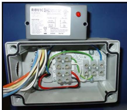
Fig. 3.15 Mounted RIB Relay
