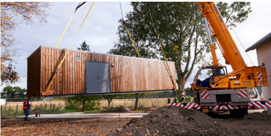
FIGURE 5: Installation of a containerized system
